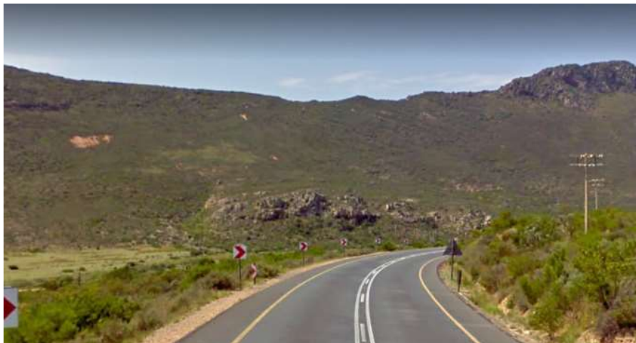
The modern R46 highway skirts Bushman’s Rock, on the left
